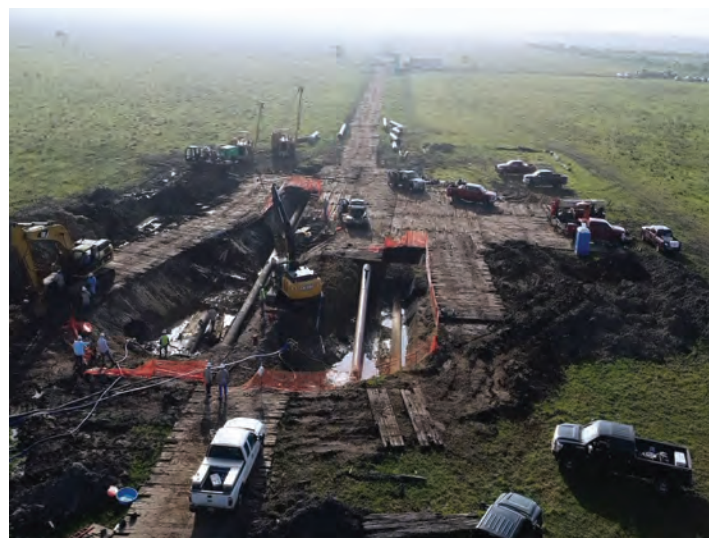
Existing pipeline relocation
