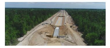
The **Luce Bayou Interbasin** Transfer Project will bring raw water from the Trinity River in a system of canals and pipelines. Construction is underway on the Capers Ridge Pump Station on the river's west bank that, when fully functional, will be able to divert up to 500 million gallons of water a day from the river, pump it into side-by-side pipelines to flow underground to a storage and sedimentation basin. Then it will flow into a canal that runs to the northeastern tip of Lake Houston.
