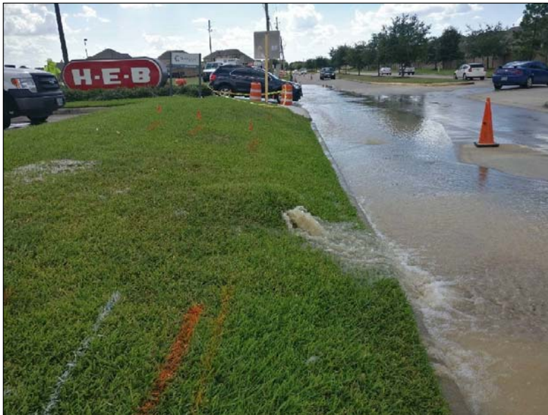
Figure 3: Water Leak
