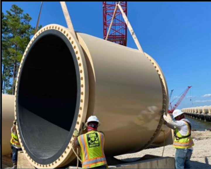
Largest (108") Magnetic Flowmeters installed in world to date
