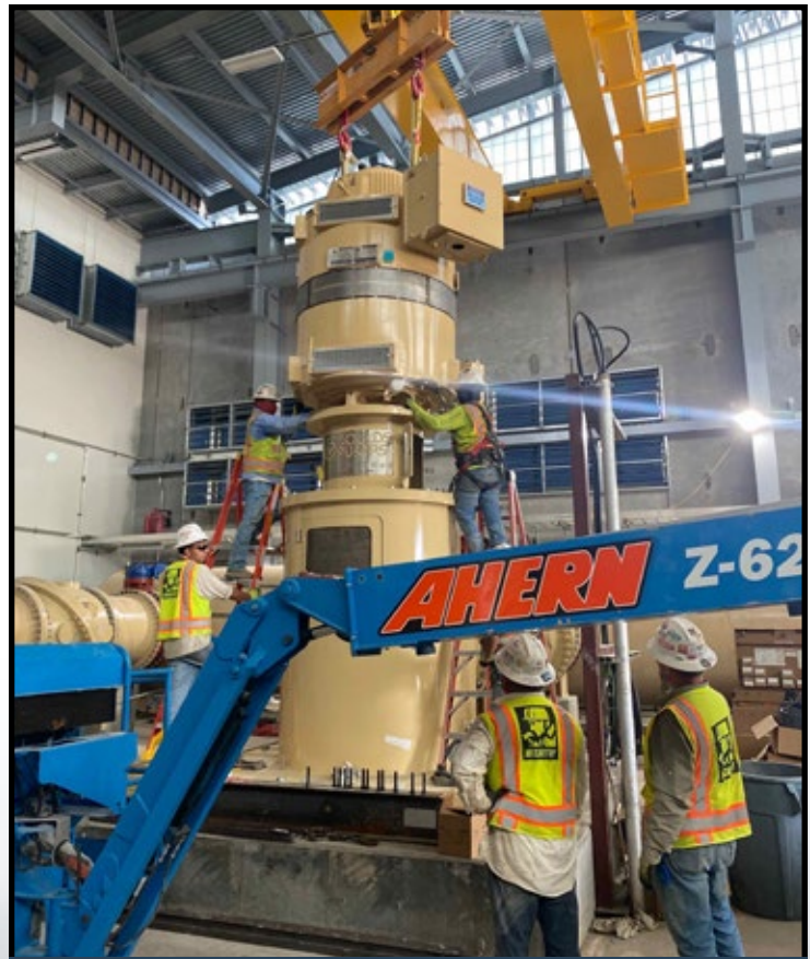
Six (6) – 1000 HP pumps are installed for a firm pumping capacity of 320 Million Gallons per Day (MGD) with room to add an additional 4 pumps for a firm pumping capacity of 560 MGD
