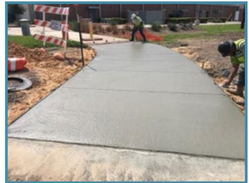
Westchase Trail Repair
