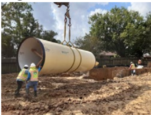
Handling Pipe within Concord Bridge
