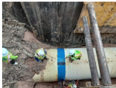
Installing Joint Wrappers
