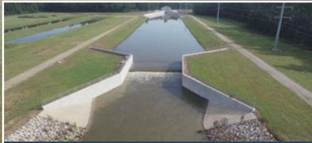
End of sedimentation basin and beginning of Luce Bayou Canal System.
