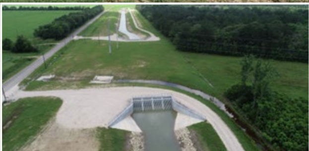
Siphon under pipeline corridor Luce Bayou Canal
