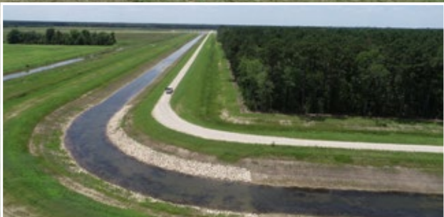
A small portion of the Luce Bayou Canal System
