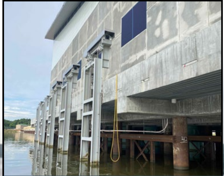
Constructed 1,000 feet off the shoreline, the intake pump station is supported by 192 – 30" Diameter piles.
