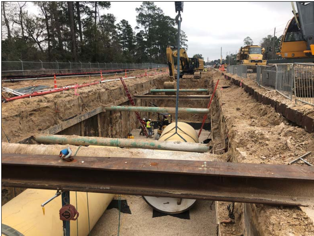
Figure 8: Laying Waterlines
