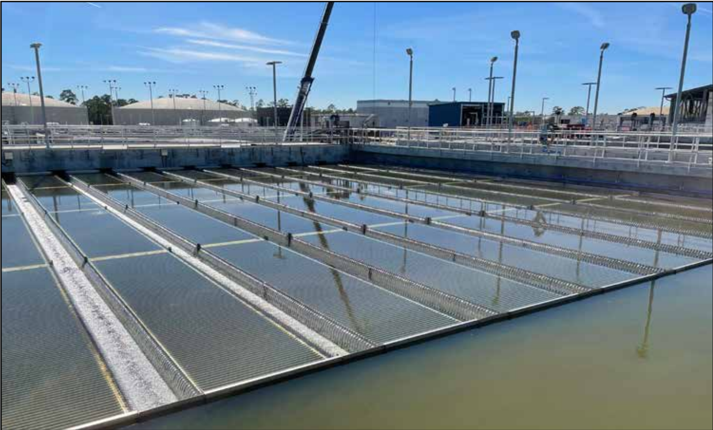
Settling Basins with Plate Settlers
