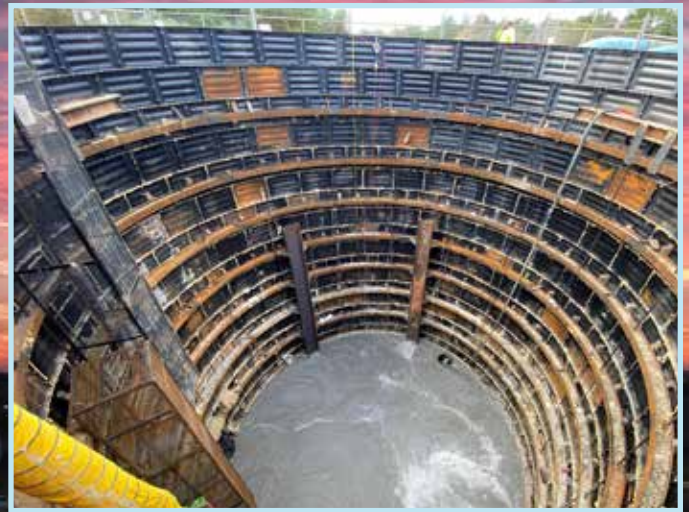
A1-A2 - Seal Slab Curing at SE Pipelines Launch Shaft
