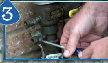
Open Test port 2. Water will continue to drain
