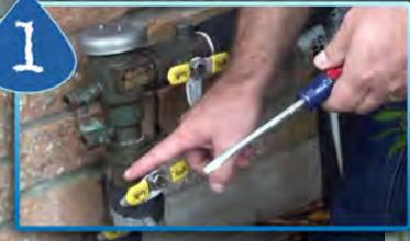
Turn the main shut off device to the off position.
